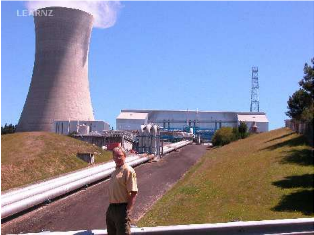
Donald standing outside the Ohaaki geothermal power station
