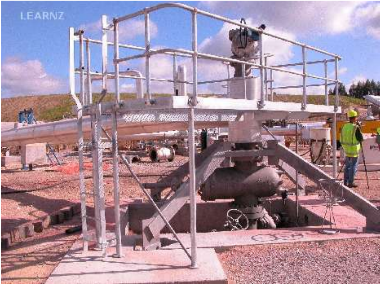
One of the four new Wairakei well heads that lie only 10 to 14m from each other.
