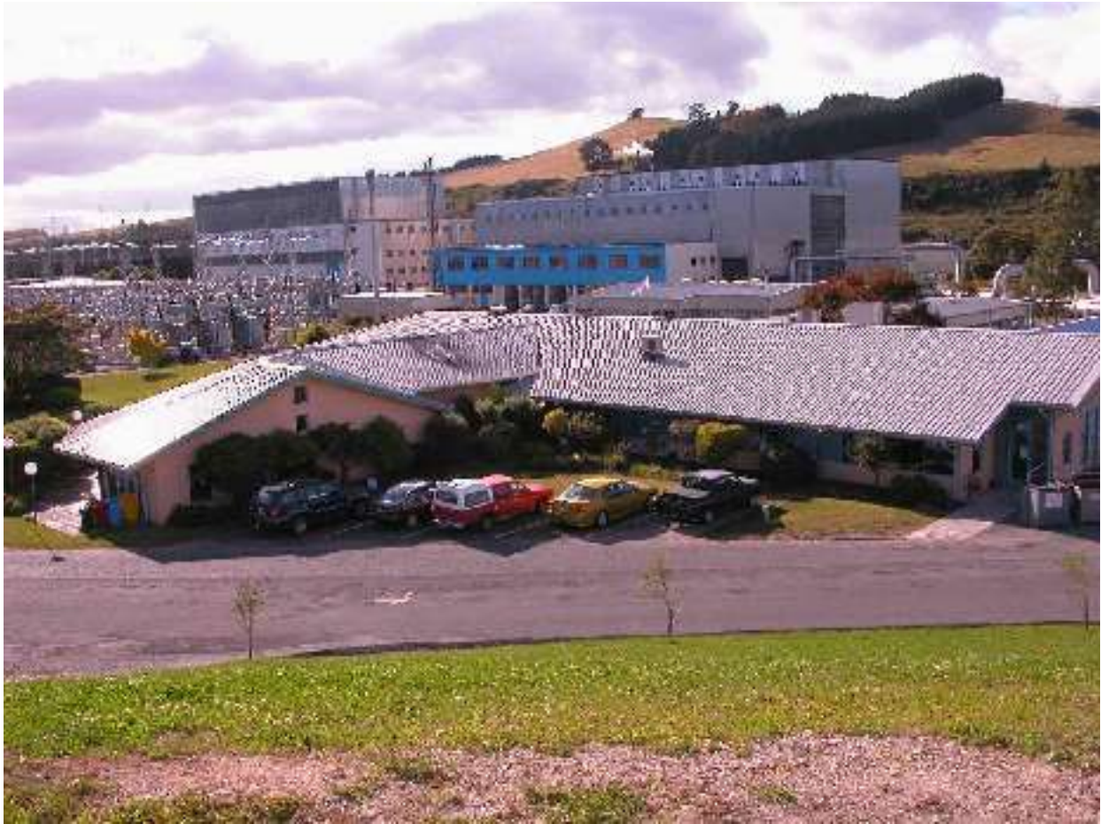
Wairakei power station. Station A is on the right and Station B is on the left. The administration centre and control room is in the foreground
