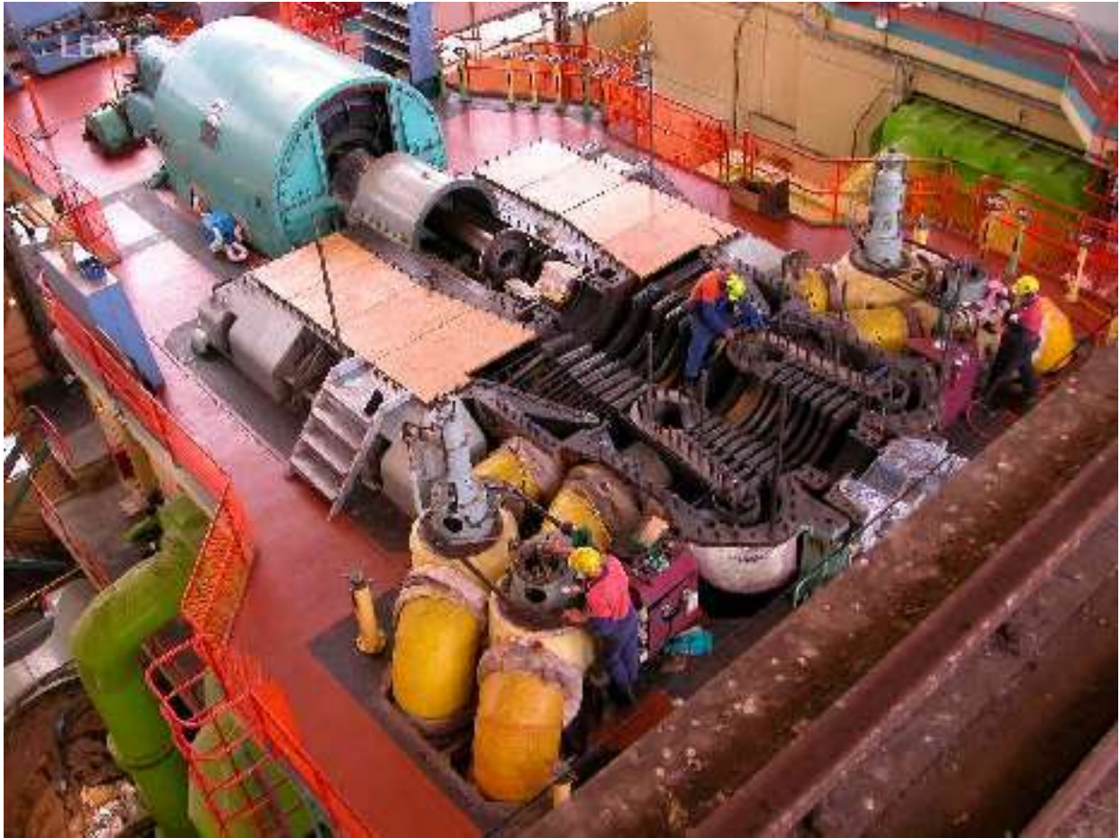
With the top casing and rotor of the MP turbine removed it is easy to see in side. The generator is green in the top left.
