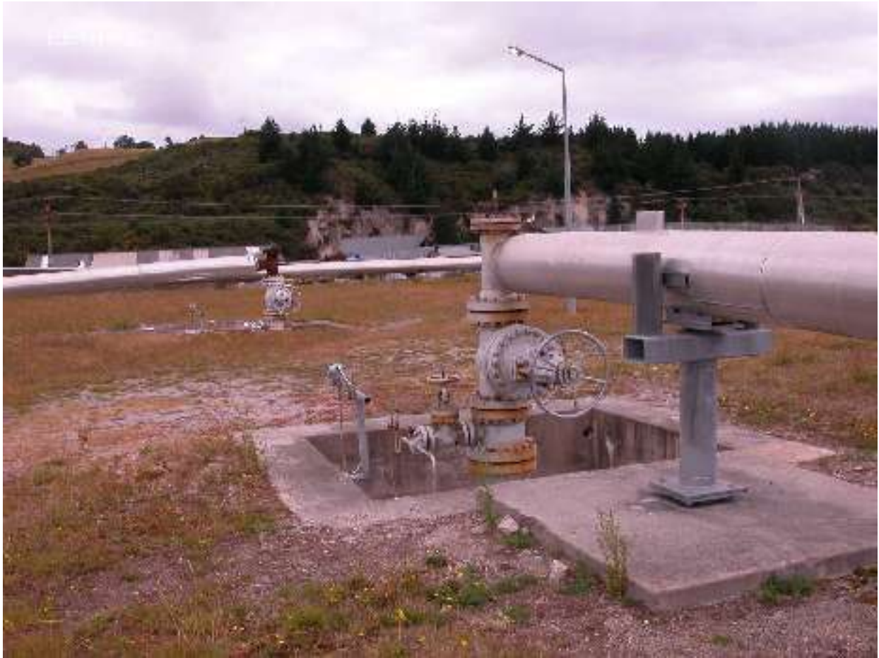
A 3km deep reinjection well near the power station. The buildings behind are part of a prawn farm which also uses waste hot water.
