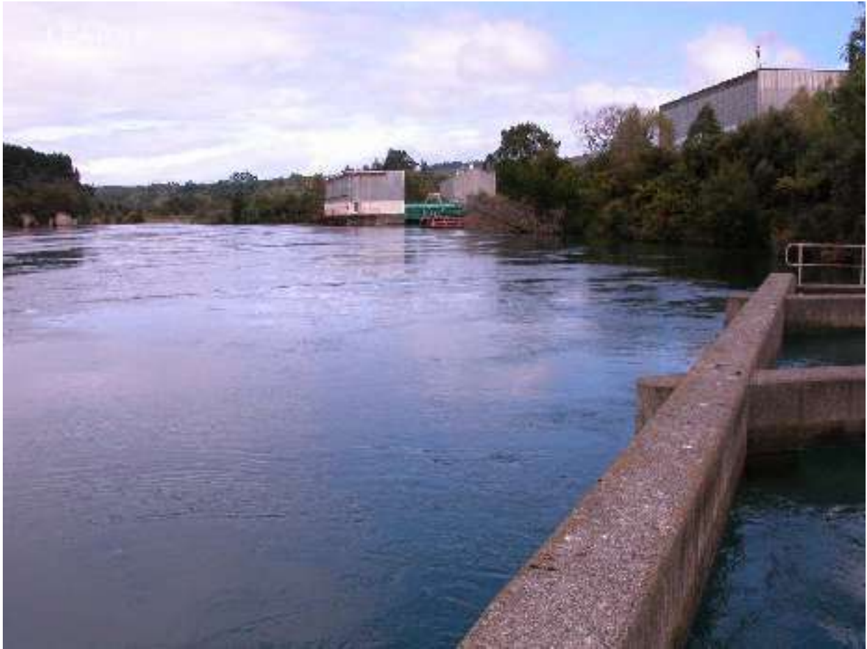
Standing on the Wairakei power station water outlet. looking up the Waikato River to the water intake building
