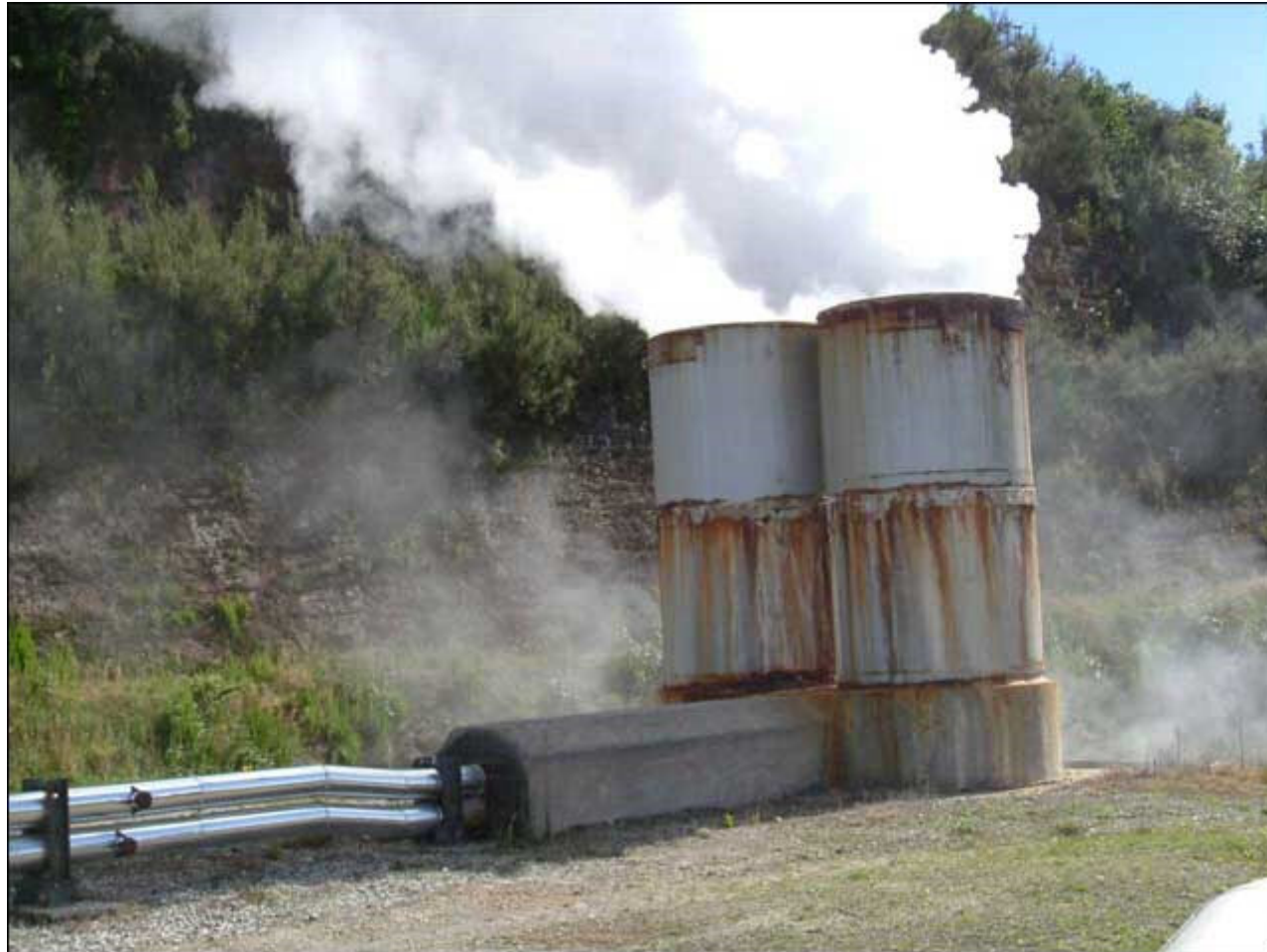
A single silencer for a single bore in the eastern borefield of Wairakei.
