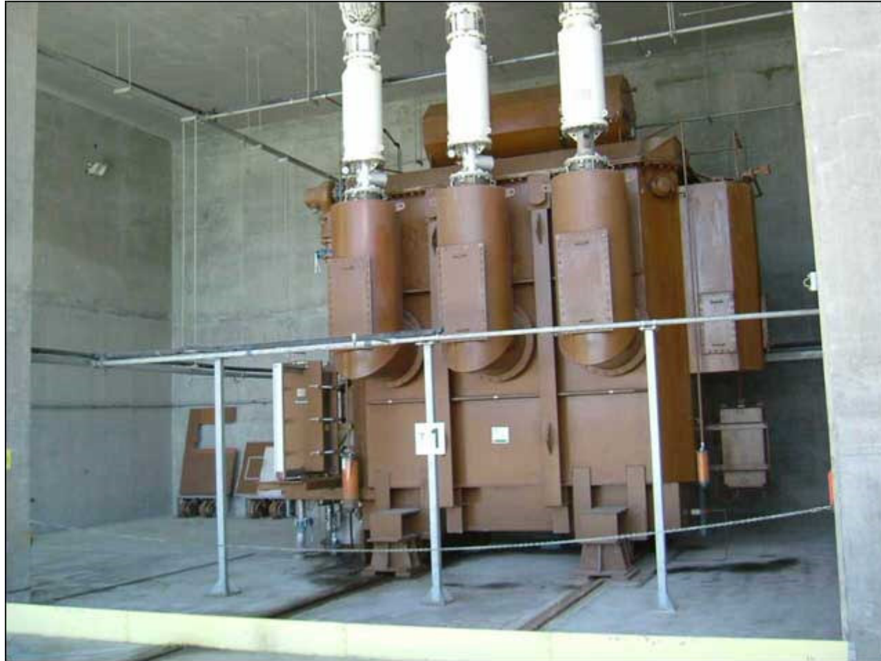
A single oil cooled transformer. Notice its ability to transform 3 phases to 220KV.
