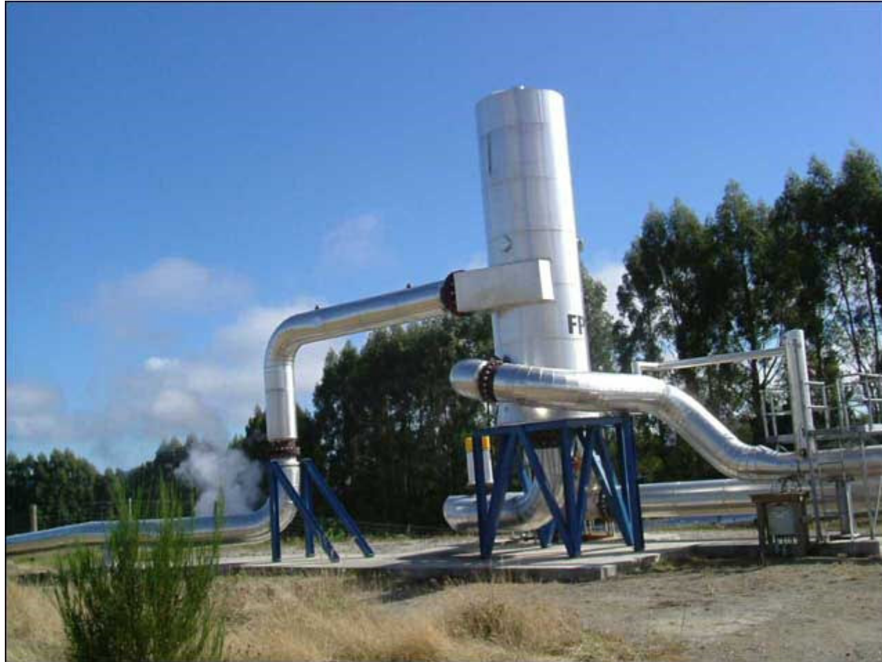
A single flash plant that services several bores.
