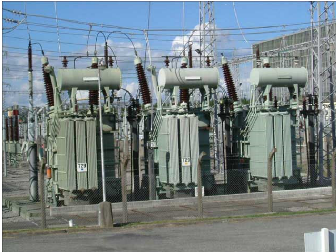
Three of the transformers in the switchyard of the Wairakei Power Station that link it to the national grid.
