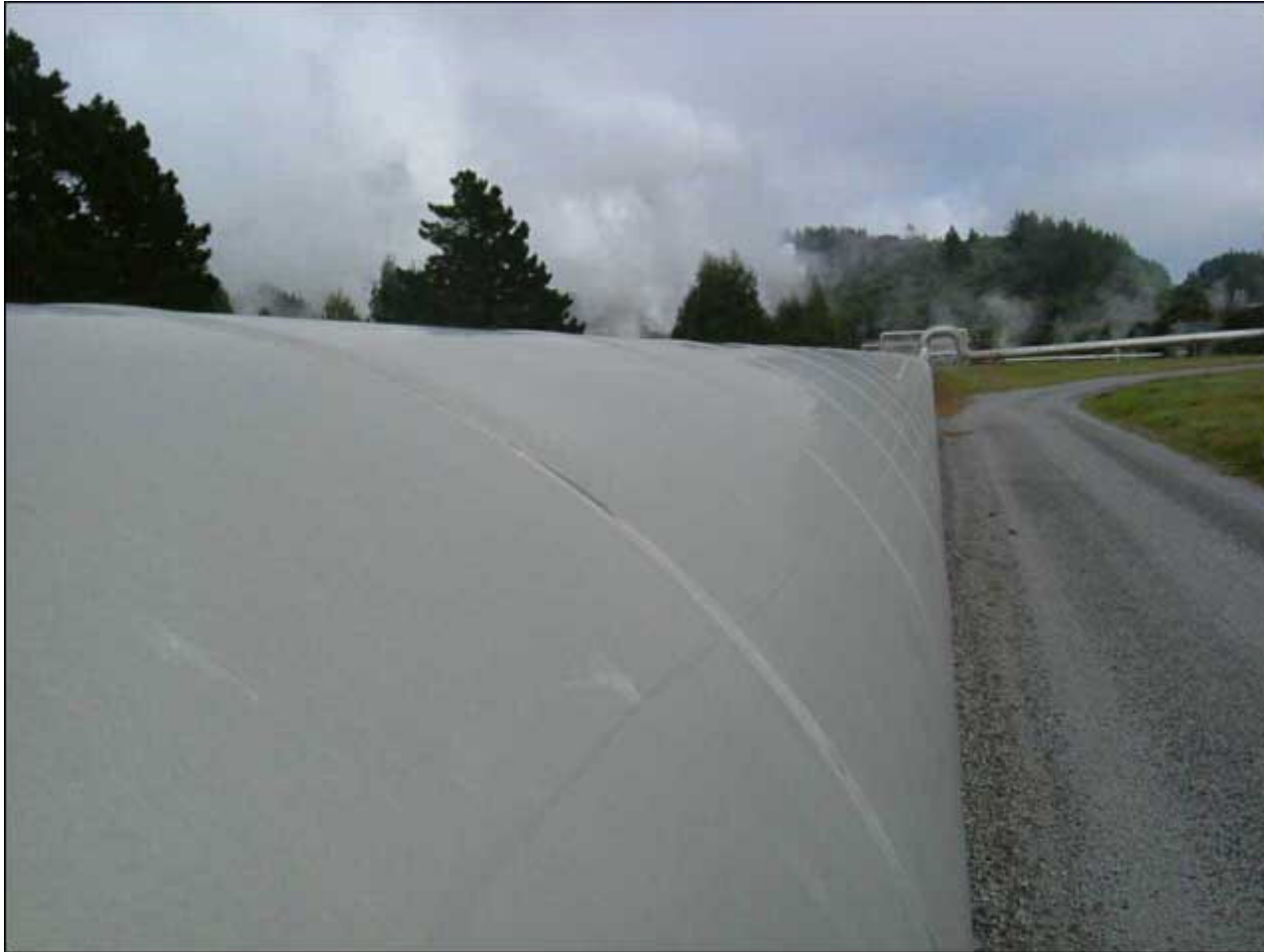
Pipeline leading from the western borefield to the Wairakei Power Station.
