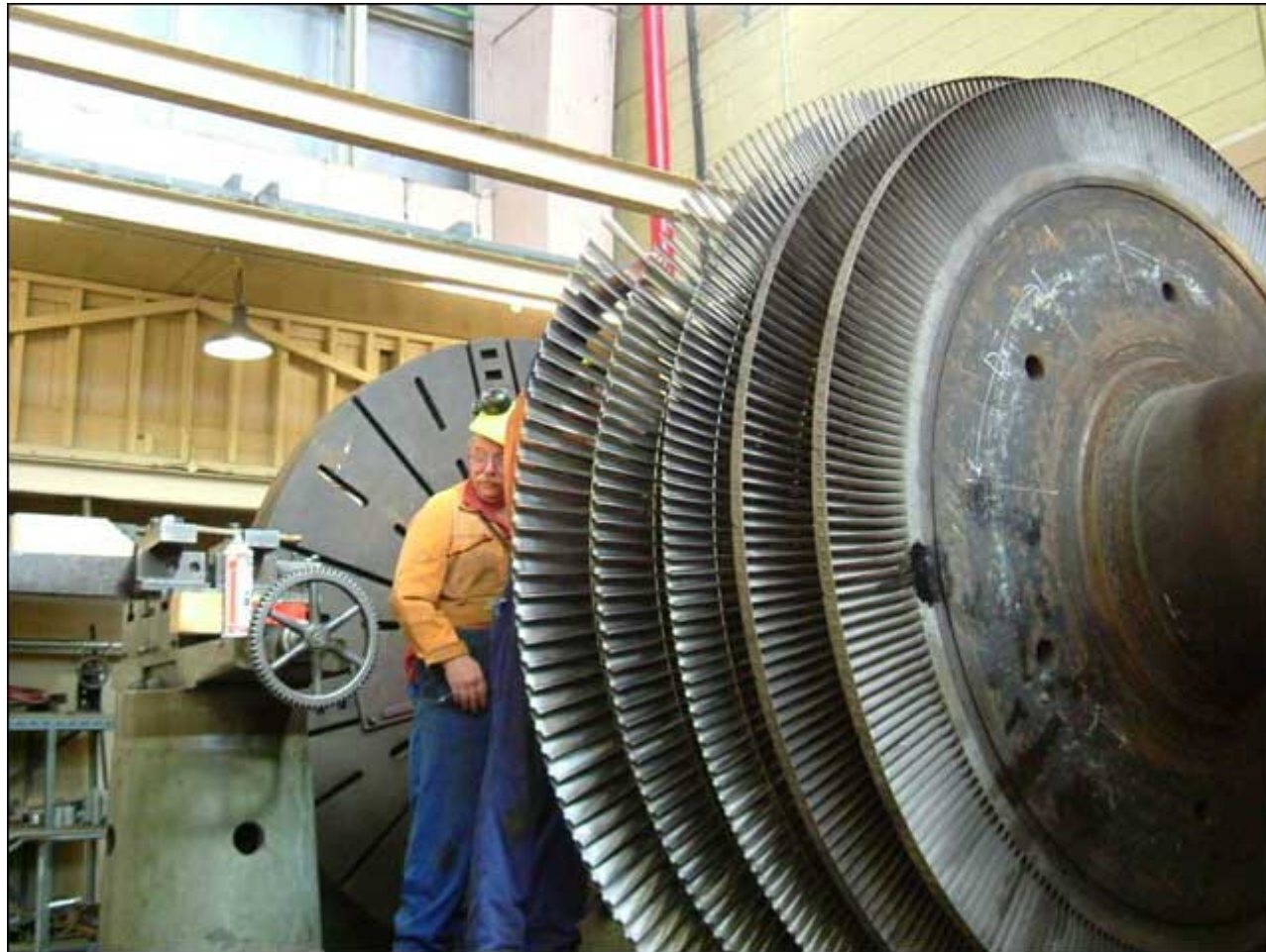
Fitting new blades to the central shaft of low pressure turbine 9. Note the 5 stages of blading.
