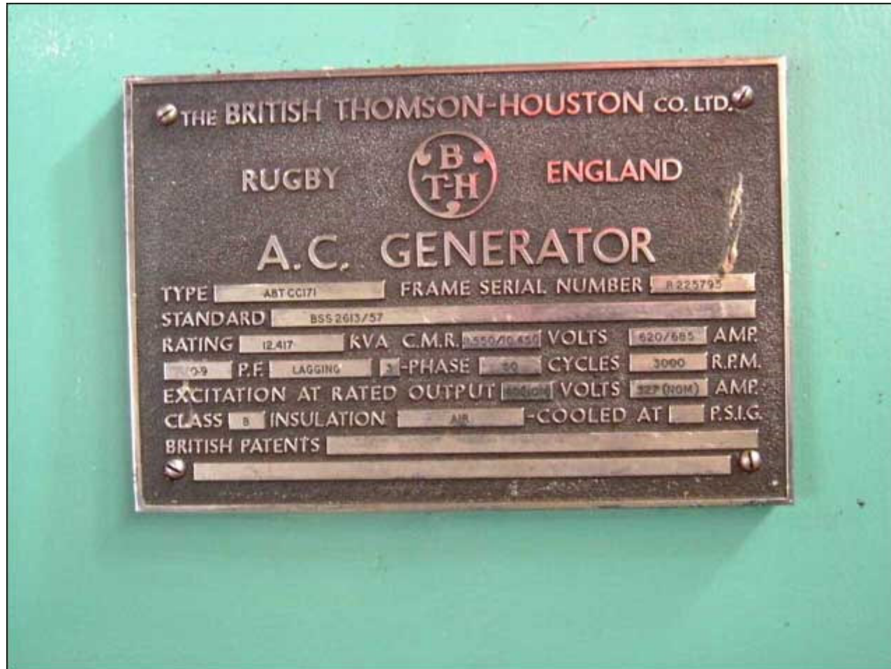
A manufacturer's plaque on Generator 4 showing the design specifications.
